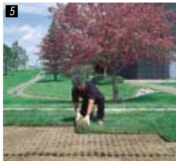
5 Hydroseed or lay sod.
